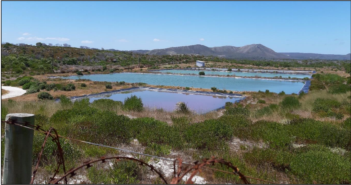
A general view of the current land-use (Eluxolweni WWTW) looking towards the east.
