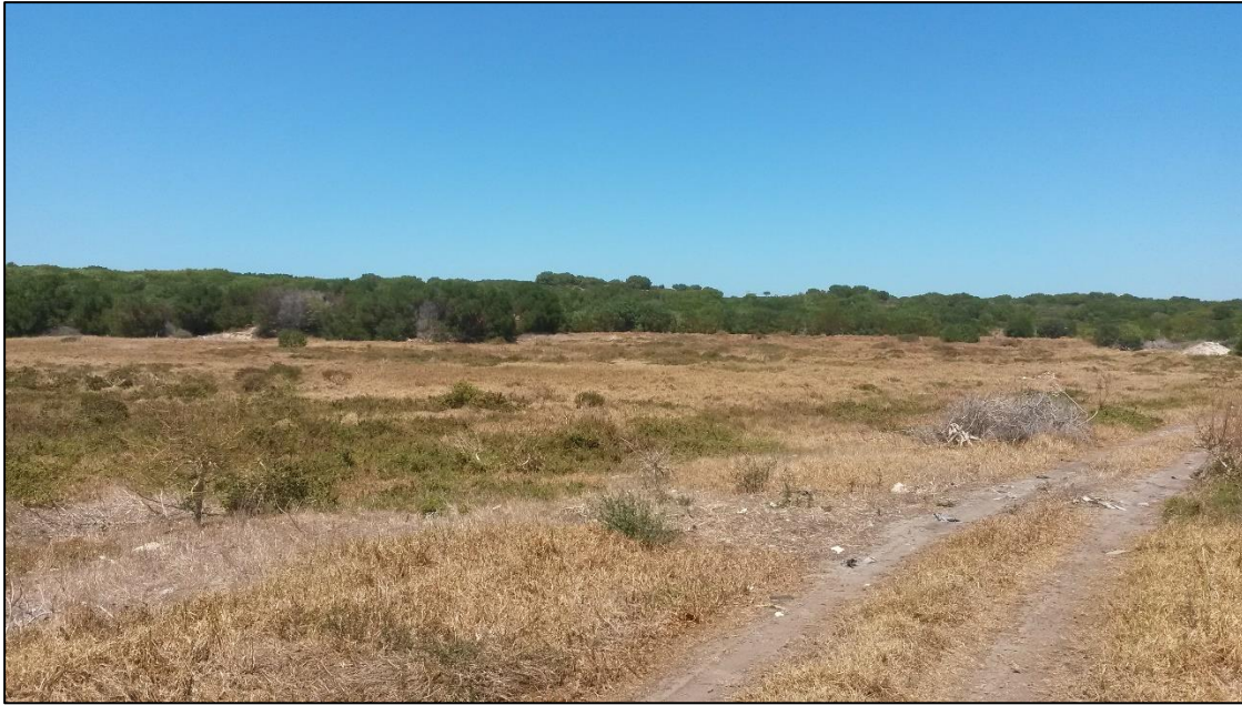
A general view of the Pearly Beach WDF in January 2015 prior to the commencement of the construction of the Eluxolweni WWTW.
